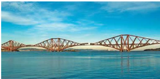
The Forth Bridge, a cantilever truss bridge
